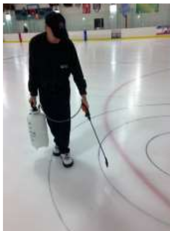
Figure 6.3: Spraying the Lines
